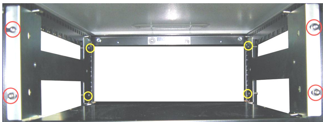
Figure 30 Installation of rack mount brackets
